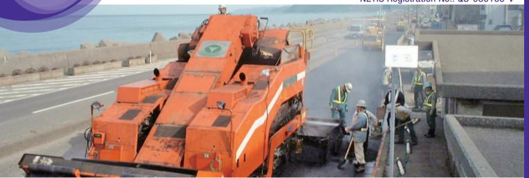
This is a pavement with excellent ability to absorb the noise generated by the road surface and tires.
